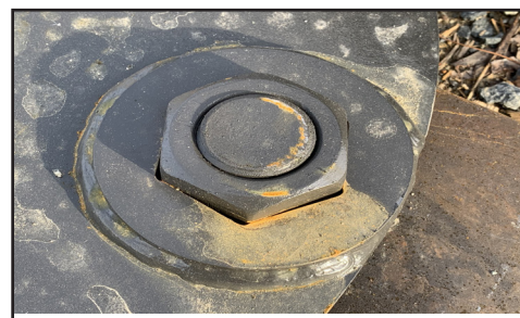
Figure 4.7b Bolt Thru Nut
